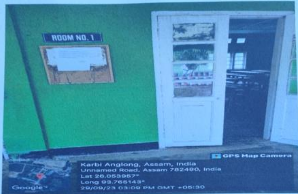
Smart class room installed on 29th May 2023 in Room-1 (Outside view)
