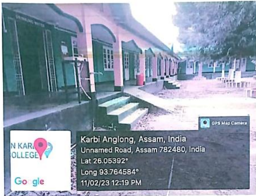
Bore well as well as rain harvested water has been distributed throughout the campus as shown in the picture above
