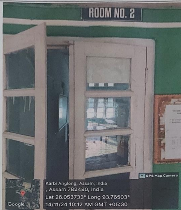
Smart classroom installed on 10/04/2023 in Room No.2 (outside view)
