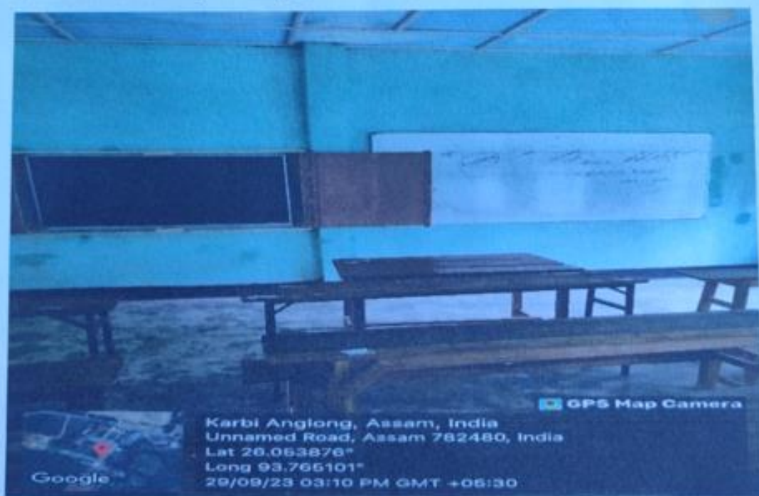
Smart class room [Room-1] (Inside view)
